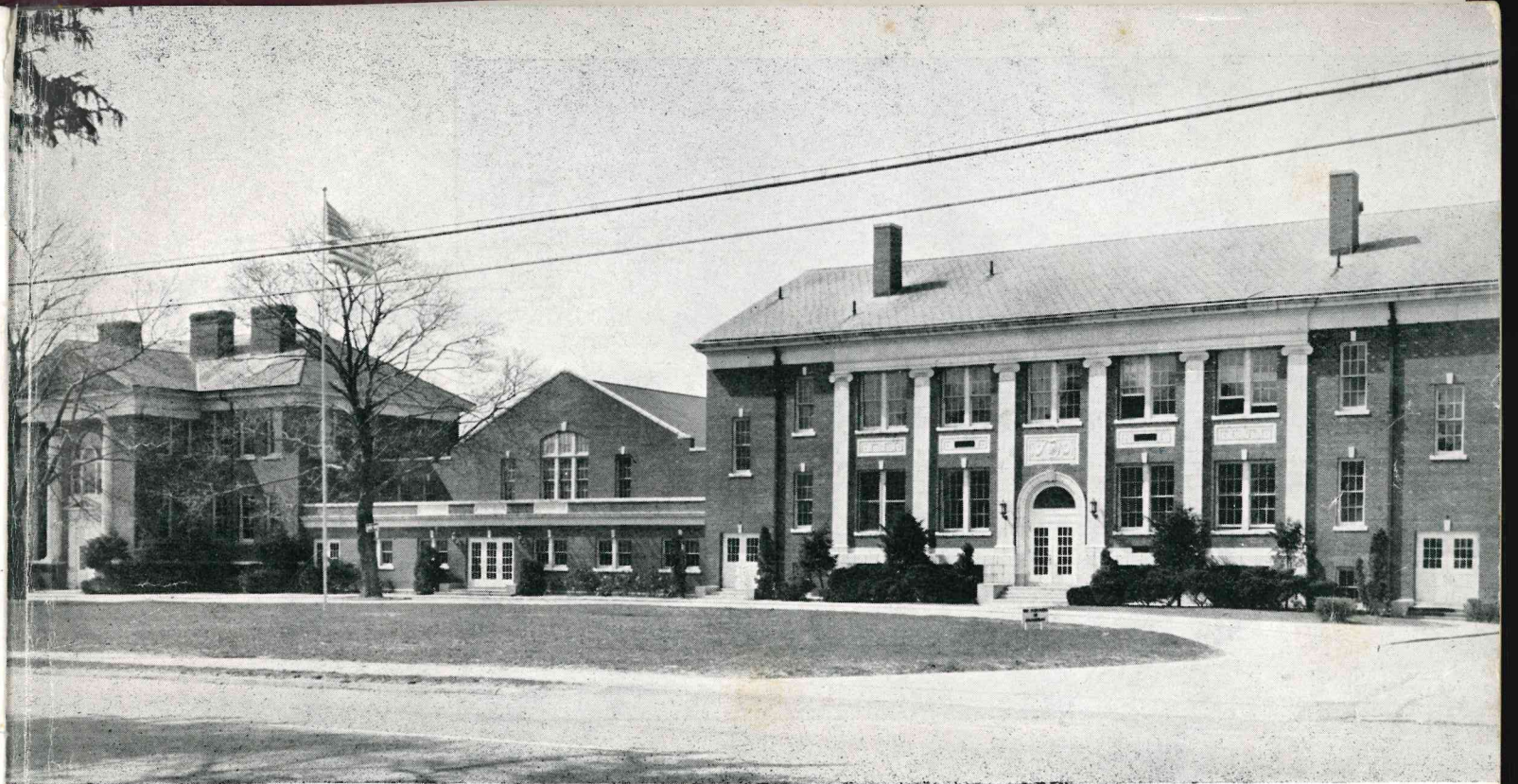
CENTRAL ISLIP HIGH SCHOOL
